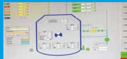
Coating Process Control Panel
